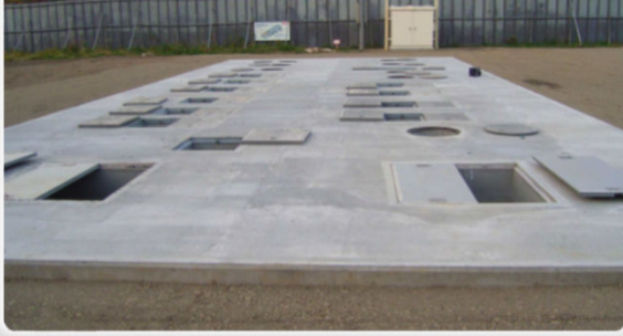
Municipal sewer project 165 m 3 /day
